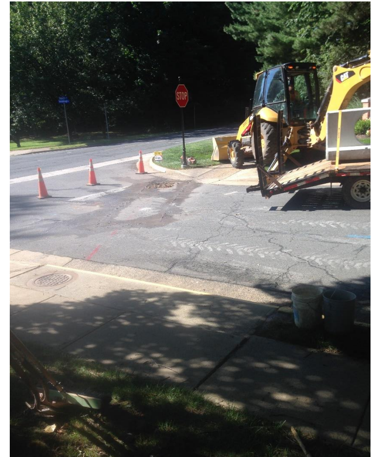
Roberts Road Entrance Storm Water Pipe Replacement
