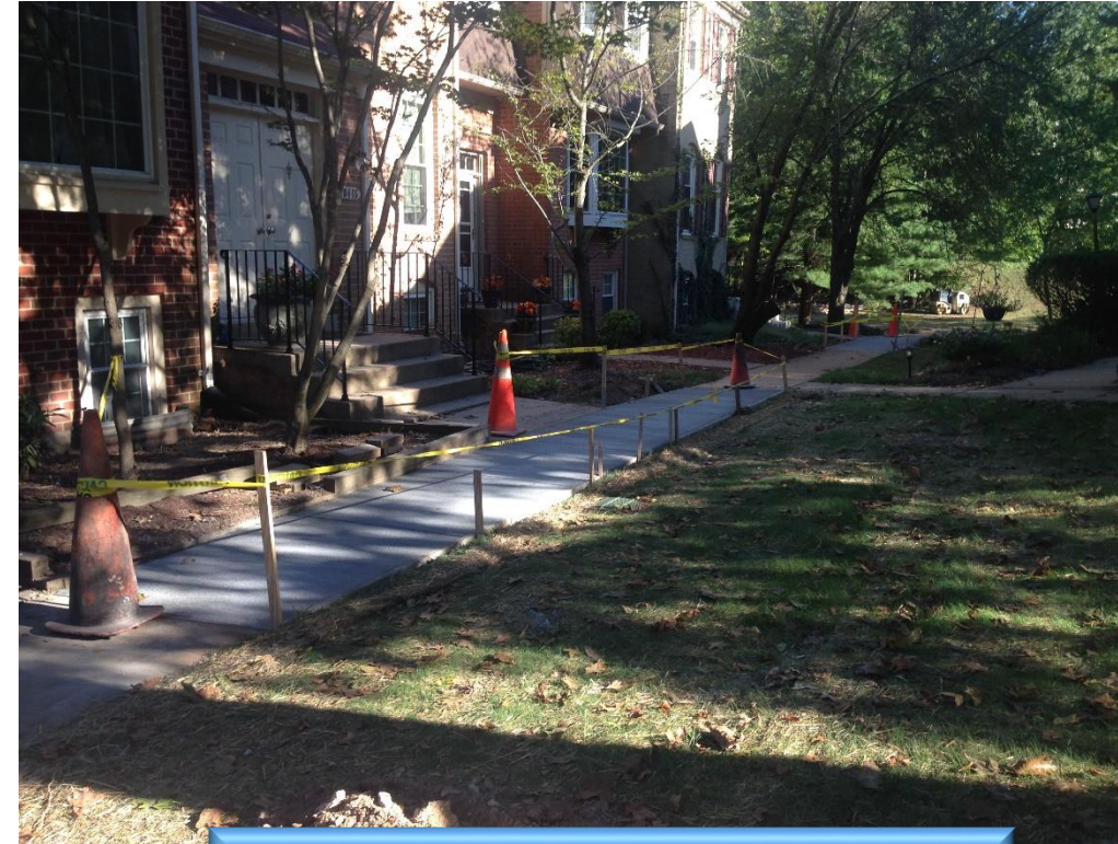
Replacement Sidewalk Sections
